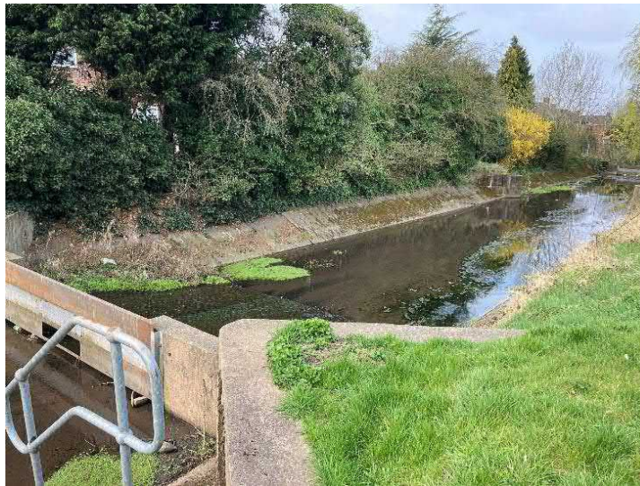
Figure 16: Site Visit Photograph - Brandhall Brook parallel to Brook Road
