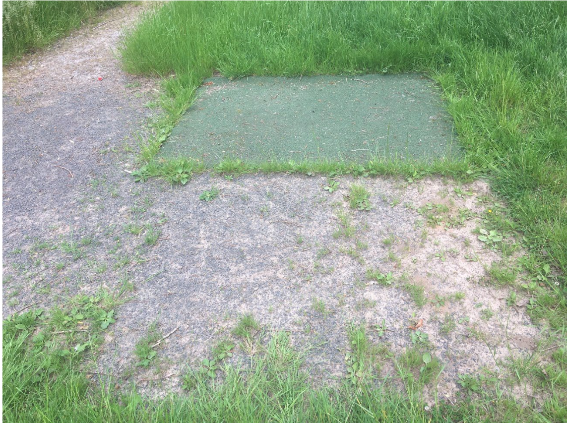
Plate 14 Surviving golf course tee and an area of concrete within the Site boundary.
